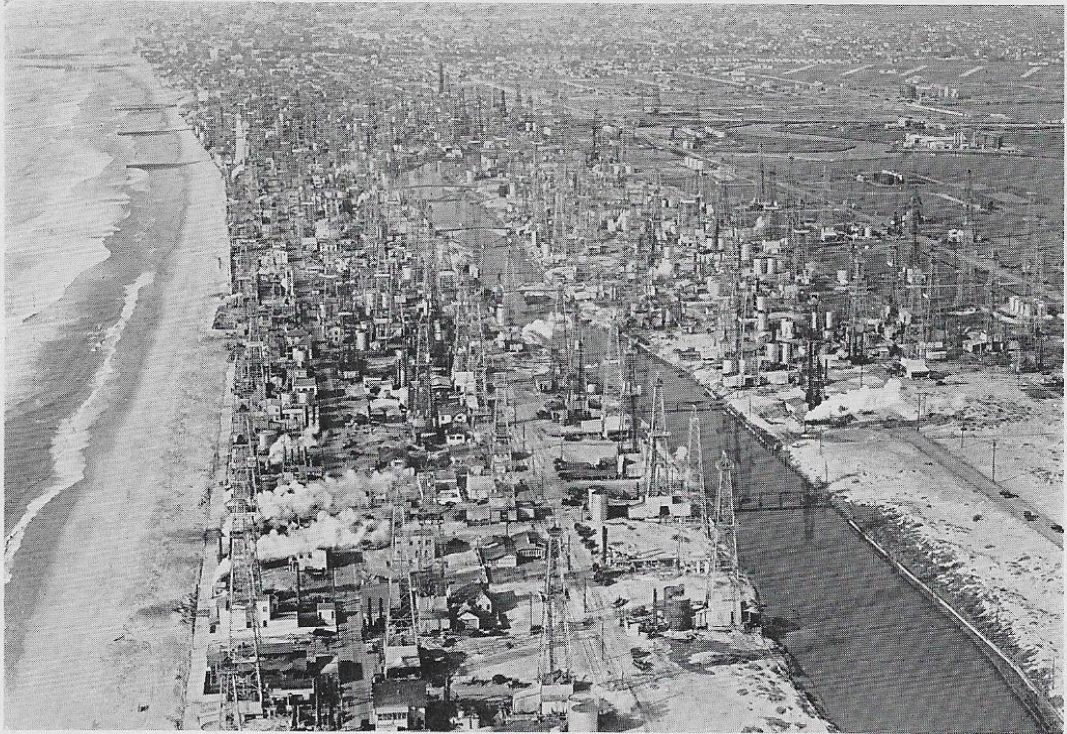
Latest view of Playa Del Rey oil field which presents one of the major curtailment problems because of tozen-lot drilling. The northwest corner of the company's big "Del Rey" lease is shown in the right foreground.
