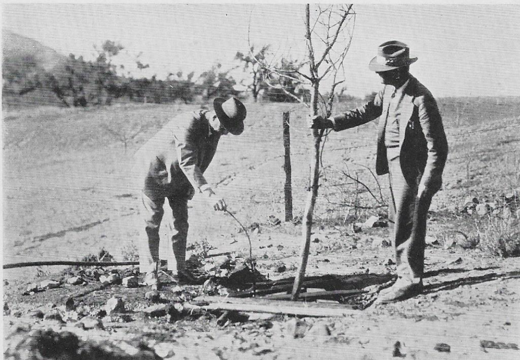
Ojai No. 6, drilled in 1865, the sixth well to be drilled in the state. It is located in Ojai canyon, five or six miles above Santa Paula. The derrick is gone, but a barrel as so of heavy oil a week oozes from the one-time well and trickles down the slope fifty yards or so before thickening into asphalt. Along the base of the hill on which Ojai No. 6 was drilled, Lewis Hardison drilled a series of 100-foot wells with a portable rig. These wells were being pumped by a single jack line when Chester Brown was assigned, in September, 1889, as a member of the crew drilling on the Astarta lease located in the canyon adjoining Ojai No. 6. In the above photograph George Gosline, superintendent at Santa Paula, is marking the old Ojai well while Mr. Brown is exploring its depths.
